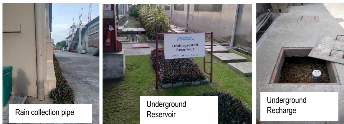
Pic 2: Catchment, Pipe networking and Storage
