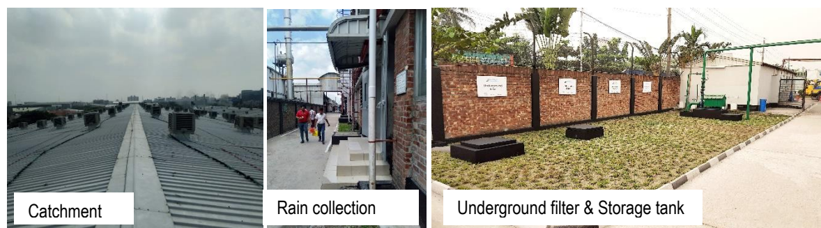
Pic 1: Catchment, Pipe networking and Storage
